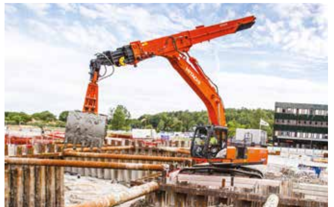
Special application excavators
